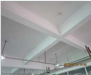
Photo of fire safety equipment Fire sprinkler and smoking detector.JPG
