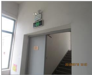
Photo of fire safety equipment Exit sign and emergency light in the dormitory.JPG
